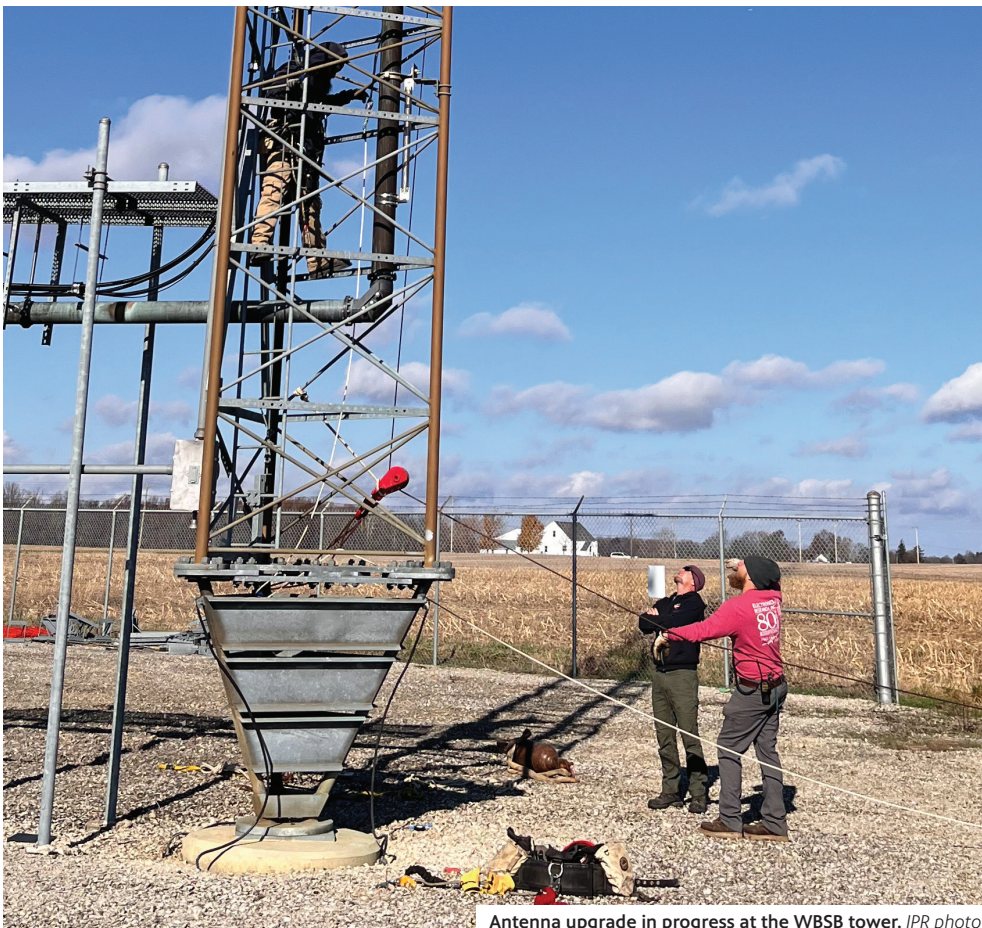
Antenna upgrade in progress at the WBSB tower. IPR photo
